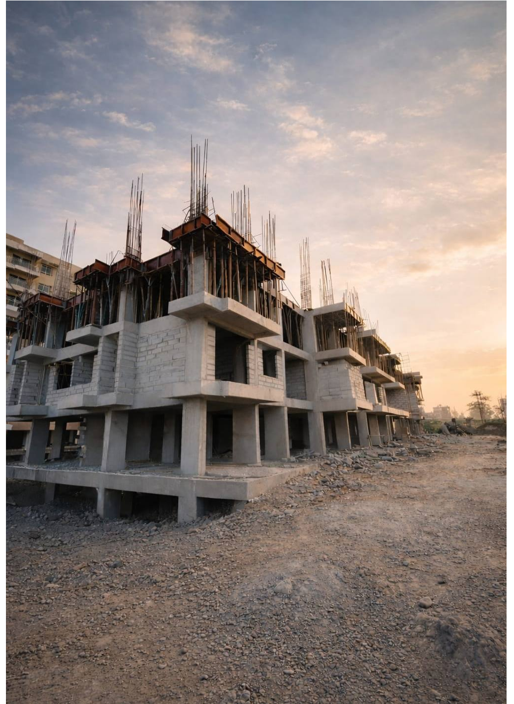
RUBY TOWER UNDER CONSTRUCTION
